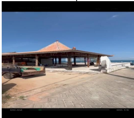
Picture 1 : The remains of the pier that have disappeared
